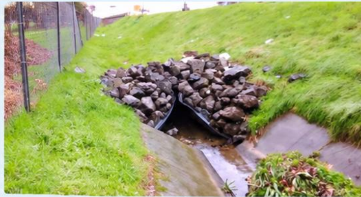
Damaged outfall
