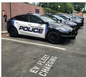
South Pasadena Police Department's all-electric patrol fleet charging on-site, demonstrating how strategic infrastructure and fleet planning enable continuous, public safety operations.
