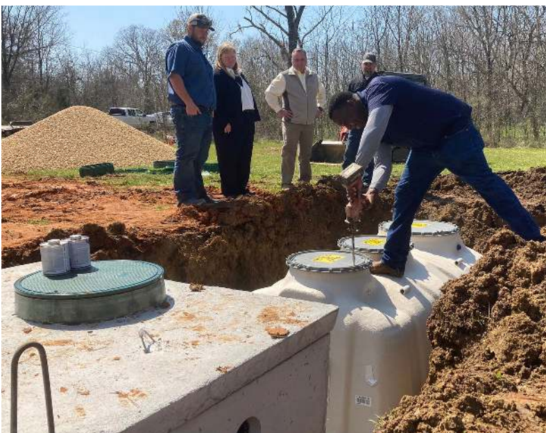
Septic Tank Installation
