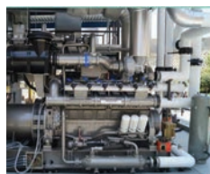
Engines supporting HCTP Cogeneration Plant
