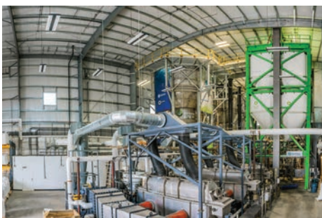
Phosphorus recovery facility, which includes Ostara Pearl reactors and the product storage/sorting silo.
