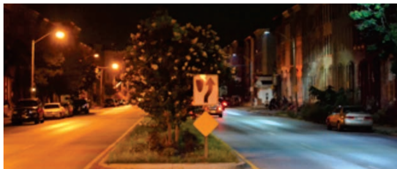
700 block of N Fulton Ave: Old fixtures on left, LEDs on right.
