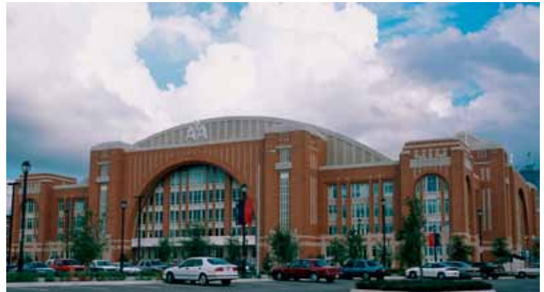
The completed American Airlines Center. (Photo provided courtesy of the City of Dallas)
