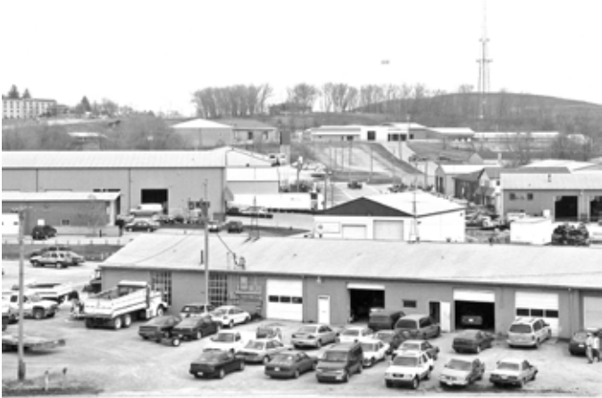
Prior to redevelopment the site was primarily industrial—encompassing more than 110 mostly underutilized or abandoned parcels owned by 74 separate individuals. (Photo courtesy of the City of Coralville)
