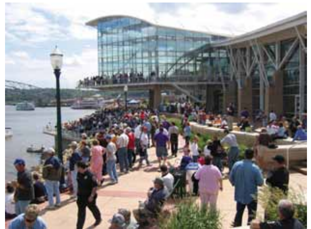
The 86,000 square foot Grand River Center is designed so that it literally seems to be cantilevered over the river. (Photo courtesy of the City of Dubuque)
