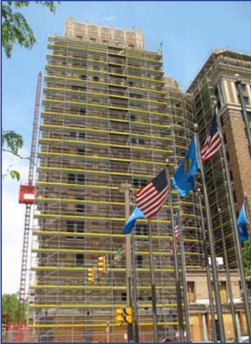
The $56 million renovation of the historic Skirvin Hotel was both extensive...
