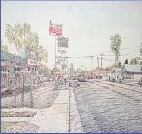
Before: an artist's rendition of Morrison Road prior to redevelopment, includes bar and scrap yard.
