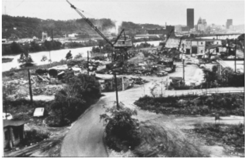
BEFORE: For two centuries, Washington's Landing was an industrial wasteland. Over the years, its 42 acres had been used for a variety of industrial operations ranging from a soap company to a slaughterhouse. (Photo courtesy Pennsylvania Department of Environmental Protection)
