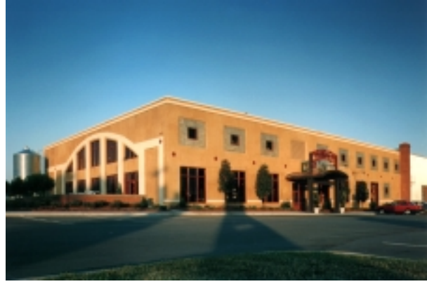
AFTER: The new restaurant has an old grain silo that was located on a Mecklenburg County farm and moved to the site. The grain silo acts as a district beacon and a billboard for the restaurant with thousands of people driving by it each day. Not only has the restaurant become Charlotte's highest grossing, it was named one of the best 10 restaurants in the country by Restaurants & Institutions magazine. (Tim Buchman Photographer)
