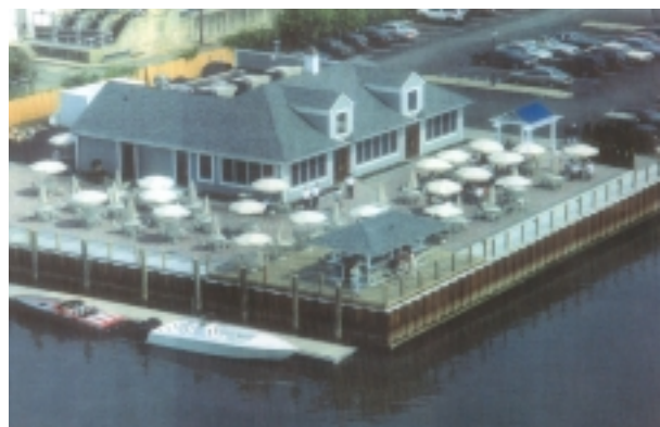
STEAMBOAT LANDING RESTAURANT: This site, on Glen Cove Creek, was formerly used as storage for landscaping equipment and materials. It is now one of the most successful restaurants in the area. This development is part of a $4M dollar private redevelopment project at the Jude Thaddeus Marina. (Photo courtesy Joe Weiser)
