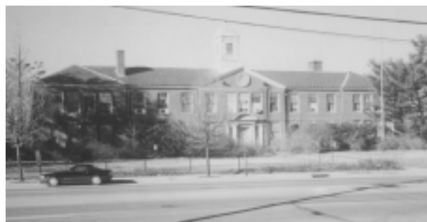
BEFORE: This school building, originally built in the 1930’s as a WP project, had been empty for years. The Glen Cove master plan slated reuse of this vacant school site as a priority. (Photo courtesy Jambhekar Strauss Architects PC)
