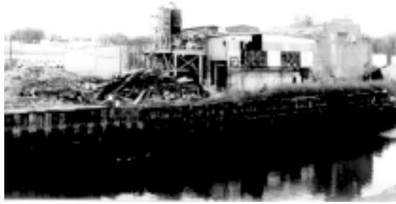
SITE STABILIZATION AT LI TUNGSTEN: This site is currently being cleaned up and is slated to be developed for cultural retail. An esplanade is being developed along this site's waterfront. (Photo courtesy Jambhekar Strauss Architects PC)
